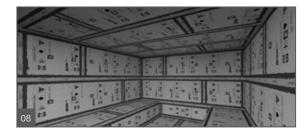
Allow the wedi Sealant 620 to cure for at least 24 hours prior to setting tile and 96 hours after its application before exposing the tiled installation to water and water vapor. On floor areas, consider wedi Fundo Shower Systems or Subliner Dry sheet waterproofing membrane when working over mortar or screed surfaces (install in accordance to Subliner Dry installation manual using wedi Sealant 620 in overlapping sheet – or Subliner Dry tape covered seam connections).
